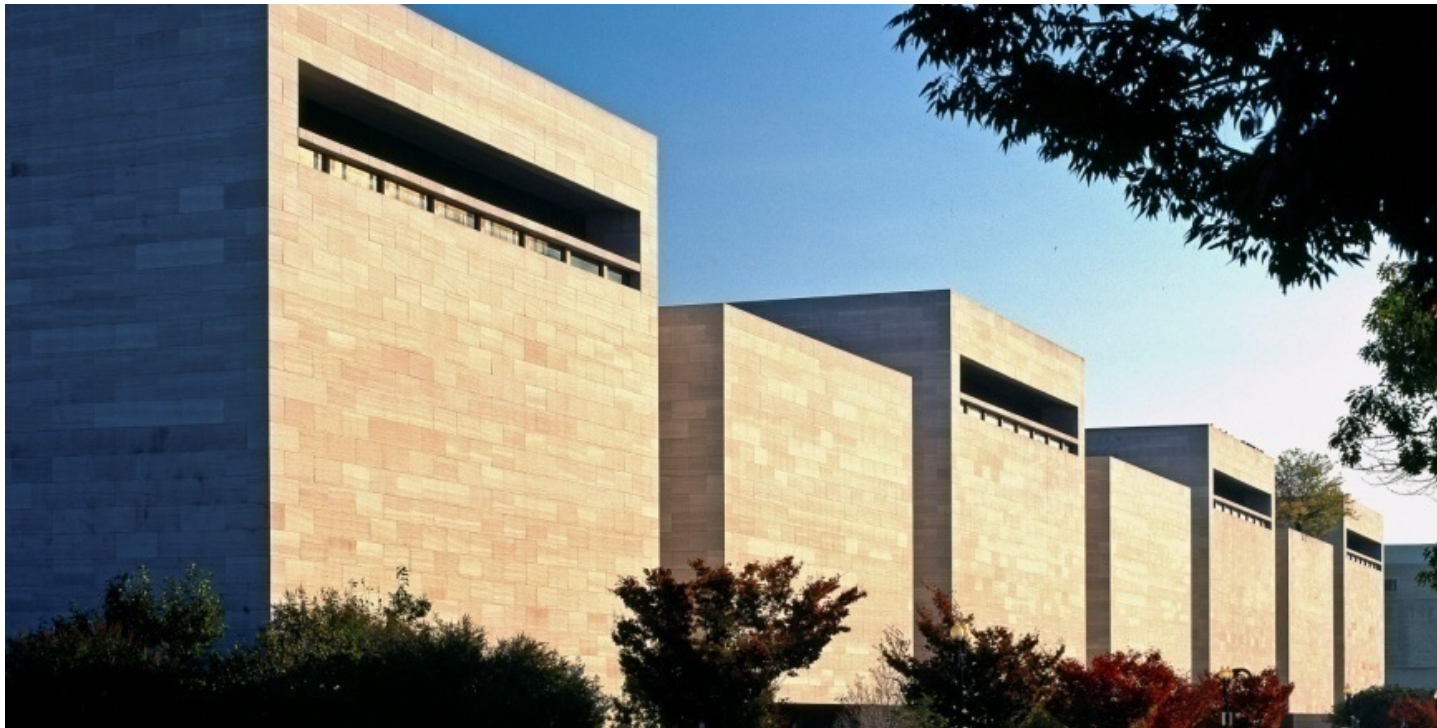
Figure 2. 9: Photo of existing building. Replacement of the stone cladding with new Tennessee Pink marble (limestone) would maintain the current visual appearance of the building to the greatest degree of any of the recladding options. (Source: QEA.)
