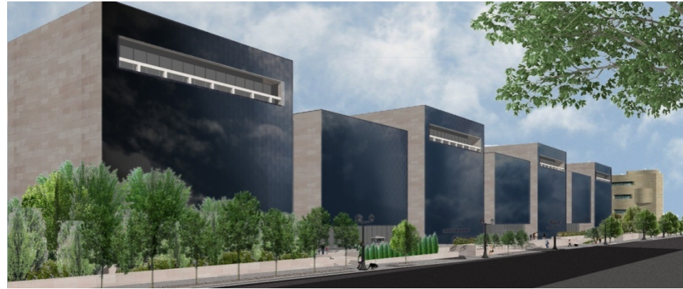
Figure 2. 47: Coplanar application of BIPV's on the entire south facade was dismissed because it was considered aesthetically oppressive and inconsistent with the volumetric massing of the original design concept. (Source: QEA.)
