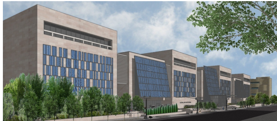
Figure 2. 48: The “Angled Plane” south wall energy harvesting concept included BIPV's interspersed with replacement stone panels, and installed on an offset frame the extended out to create a canopy that offered shade at the plaza level. This option was dismissed because the panels created a form of ornament that would distract from the originally intended simple massing of the building. (Source: QEA.)
