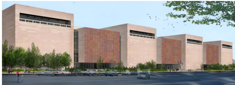
Figure 2. 50: Terra cotta colored BIPV's on the partial height pavilions alternate with the stone cladding to be applied on the adjacent full height pavilions. This option was dismissed because the planar application was too much of a departure from the volumetric massing of the original design concept and the terra cotta color was incongruous with the adjacent cladding. (Source: QEA.)
