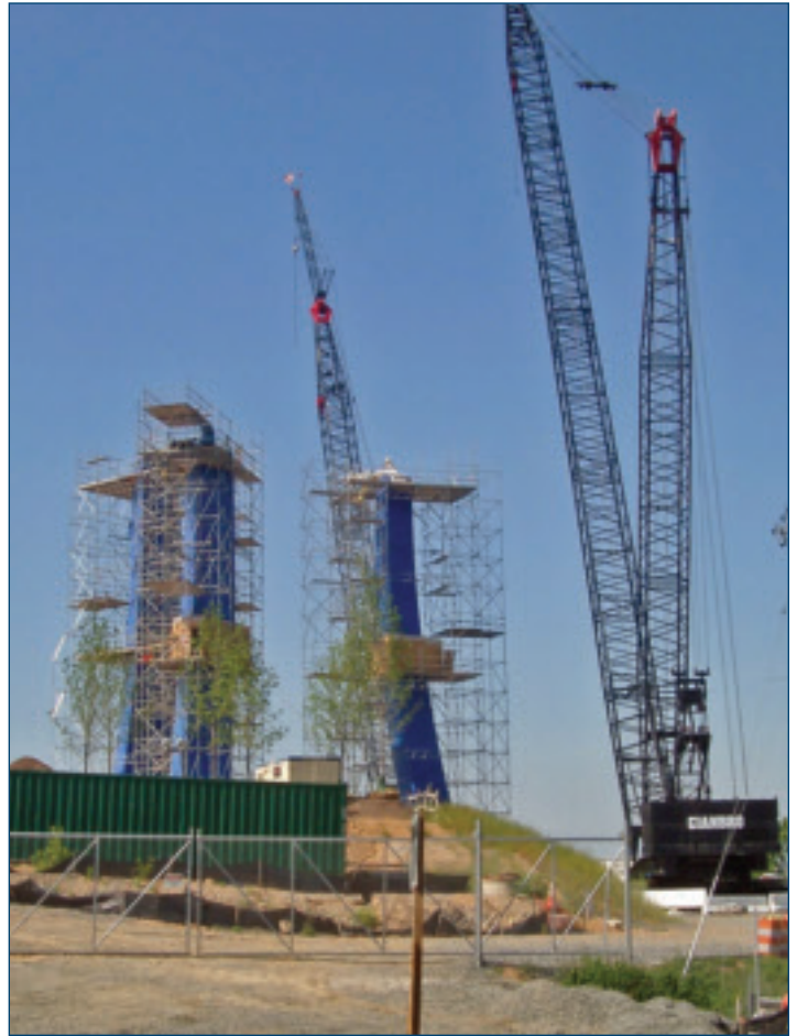
Fig. 10 — During the erection phase, 40-ft sections were successfully welded together. The blue outer wrapping protects the exterior finish. (Photo courtesy of Avesta Welding, LLC, Ron Stahura, photographer.)
