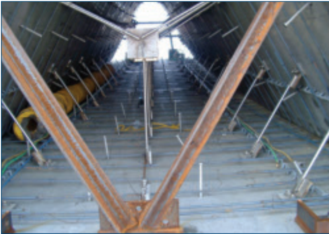
Fig. 5 — The interior of a modular section showing stiffeners that were welded to the anchor studs. (Photo courtesy of Avesta Welding, LLC, Ron Stahura, photographer.)
